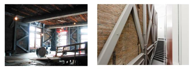
Figure 2. Structural steel seismic bracing – Canadian Museum of Nature, Ottawa. [3]
